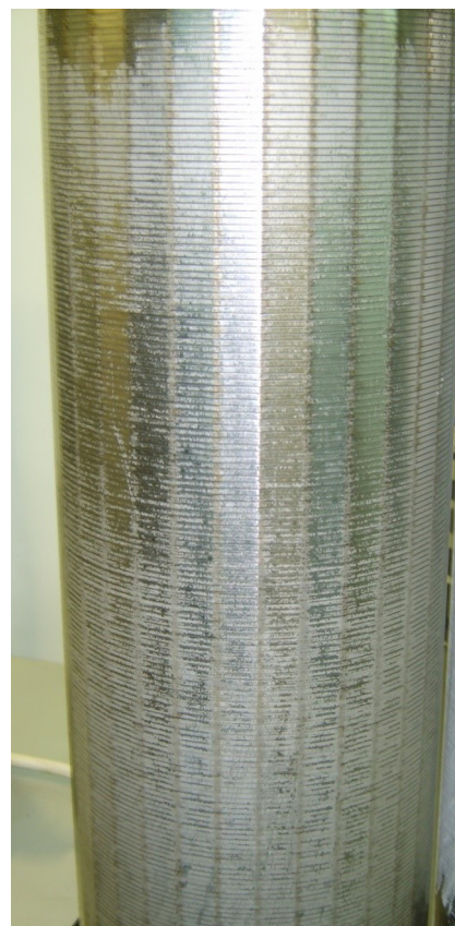
Fig. 9. Filter tubes in the test wells.
