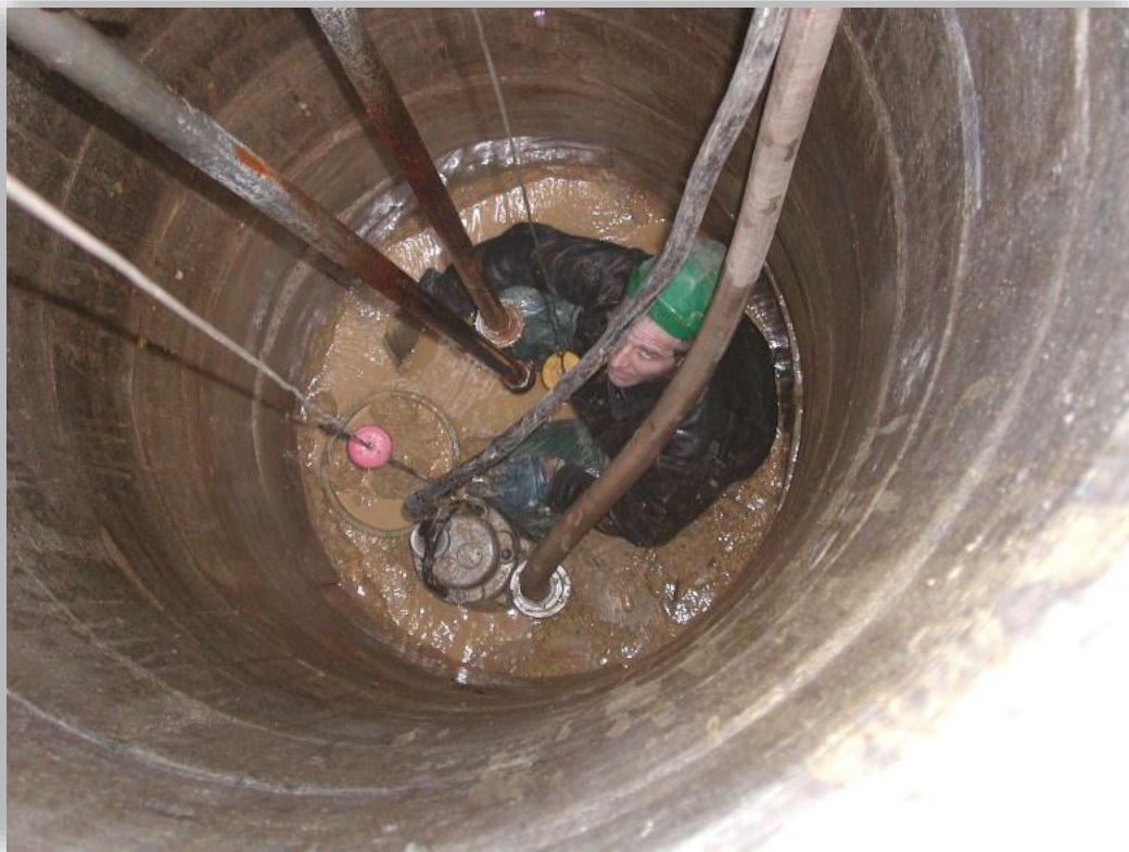
Figure 6.1 Rehabilitation of cleaning of well at Radouň, Czech Republic
