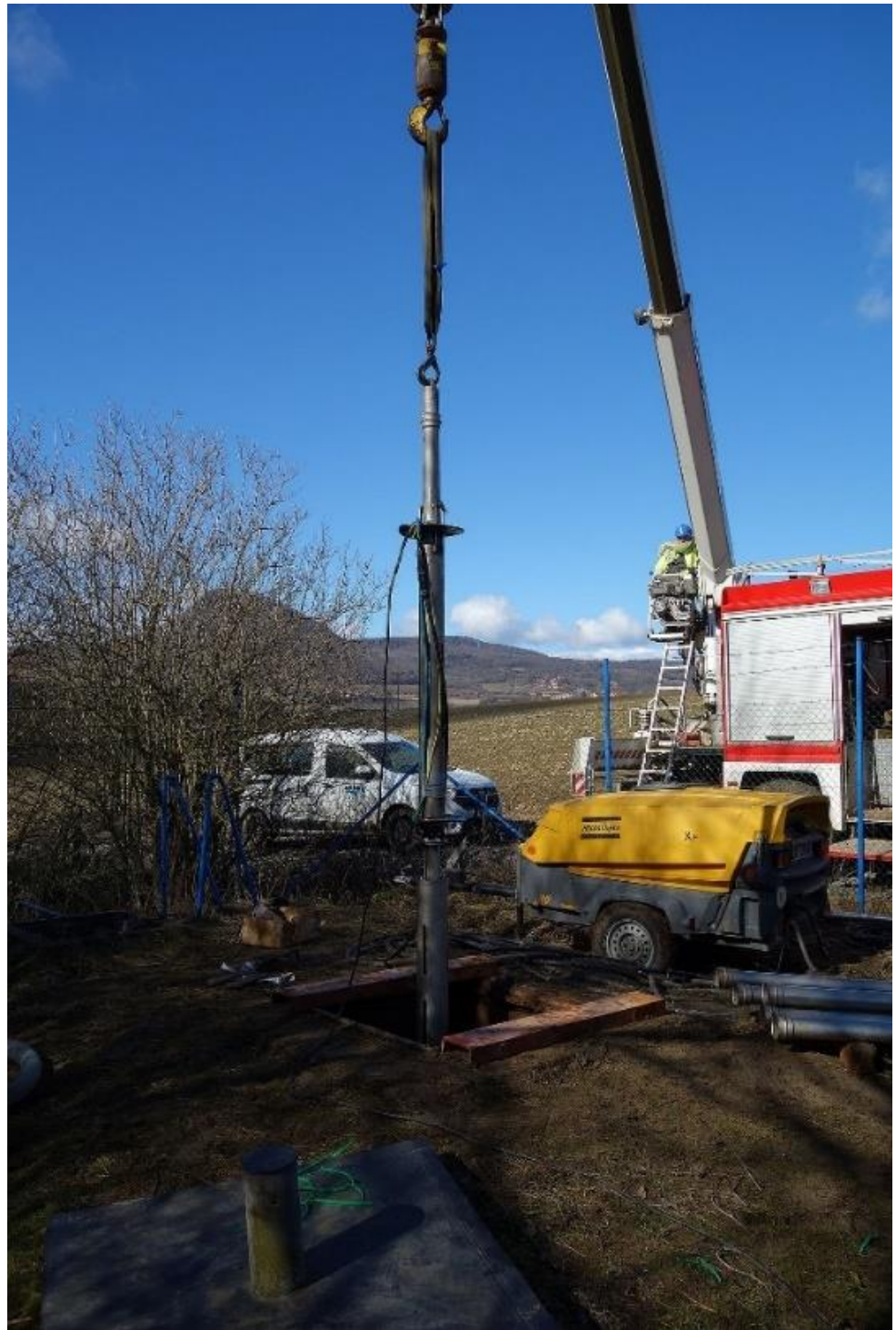
Figure 7. Rehabilitation set built within the project.
