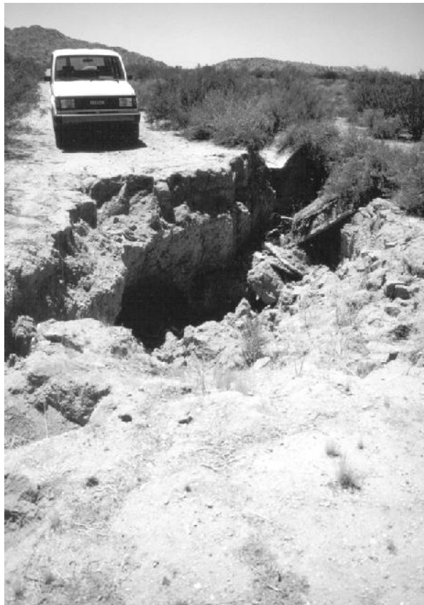
Figure 5.12 Upper photo: aerial view of a fissure in the Picacho Basin near Eloy, Arizona. The fissure stands out due to the vegetation in it. In the background are a road and cultivated fields. Photo copyright of Larry D. Fellows, Arizona Geological Survey; reprinted with permission. Lower photo: recent fissure cutting a dirt road in the Higley Basin near Phoenix, Arizona. Photo copyright of Raymond C. Harris, Arizona Geological Survey; reprinted with permission.
