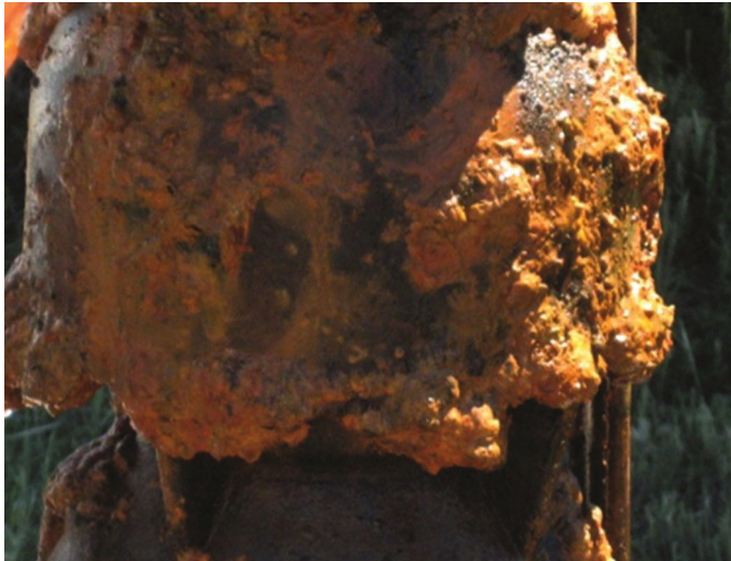
A submersible pump being pulled from a well exhibiting iron oxide, iron bacteria and biofilm.
