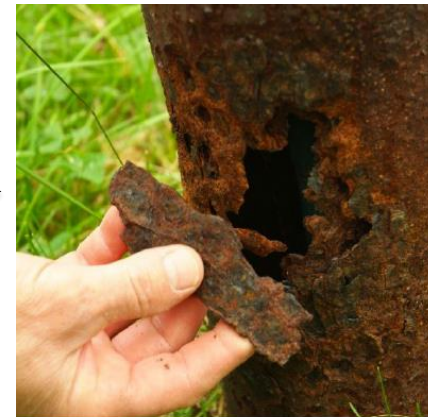
Hole in casing caused by corrosion
