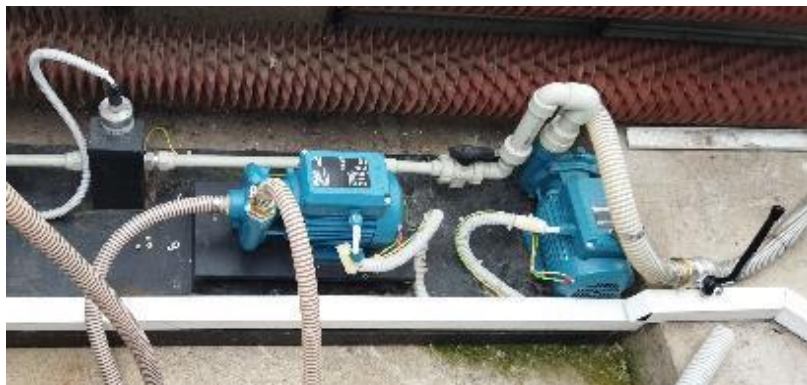
Figure 4. Placement of Calpeda C 20E 230V circulating pumps
